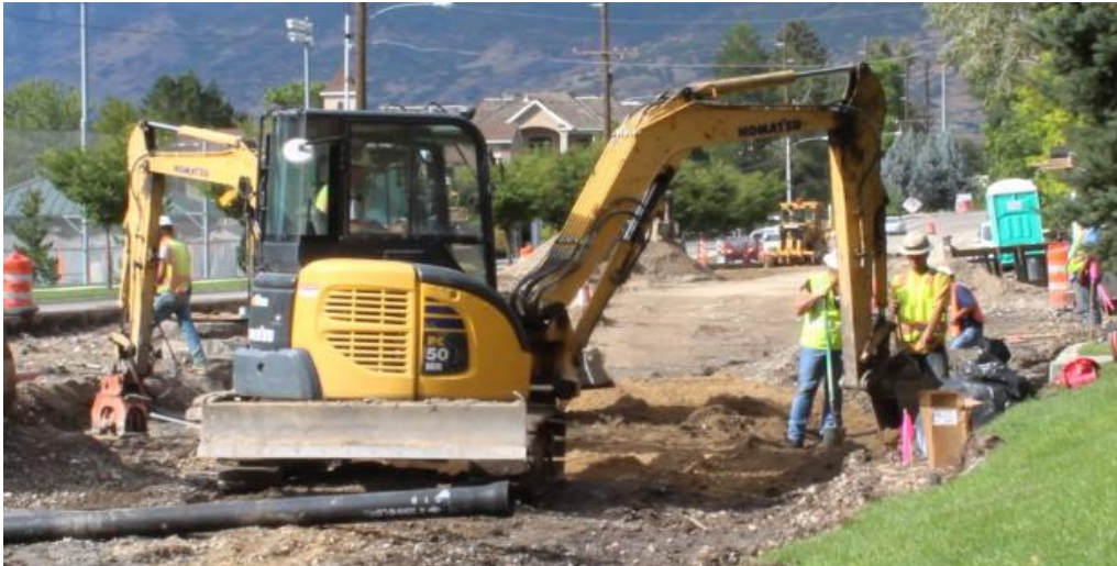
Fig. 7. Clearing of site work
