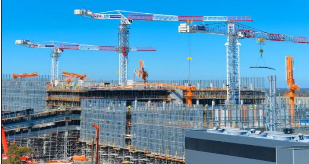
Fig. 5. Cranes on construction site
