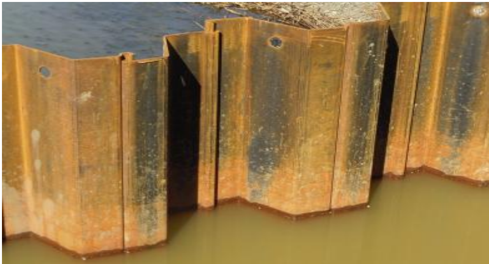
Fig. 10. Sheet pile walls [9]
