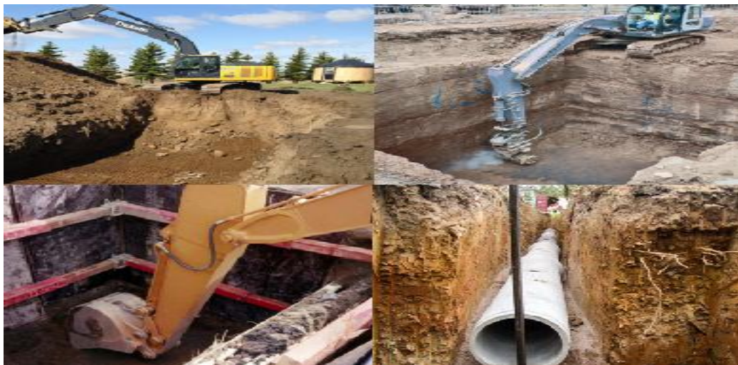
Fig.4. Excavations of piles, basement, foundation and manhole
