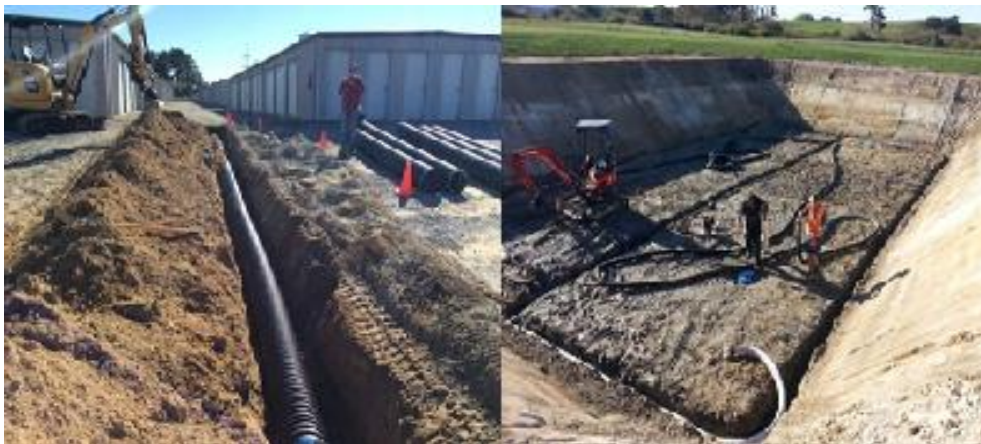
Fig. 8. Control drainage system on site work
