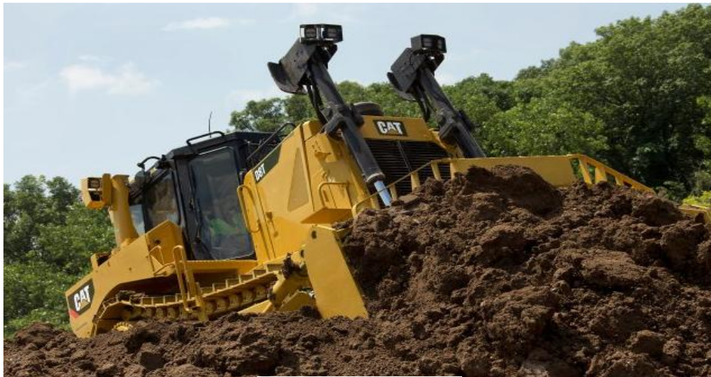
Fig.3. Cutting soil by dozer
