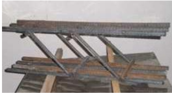
Fig. 1: Typical welded swimmer bars
