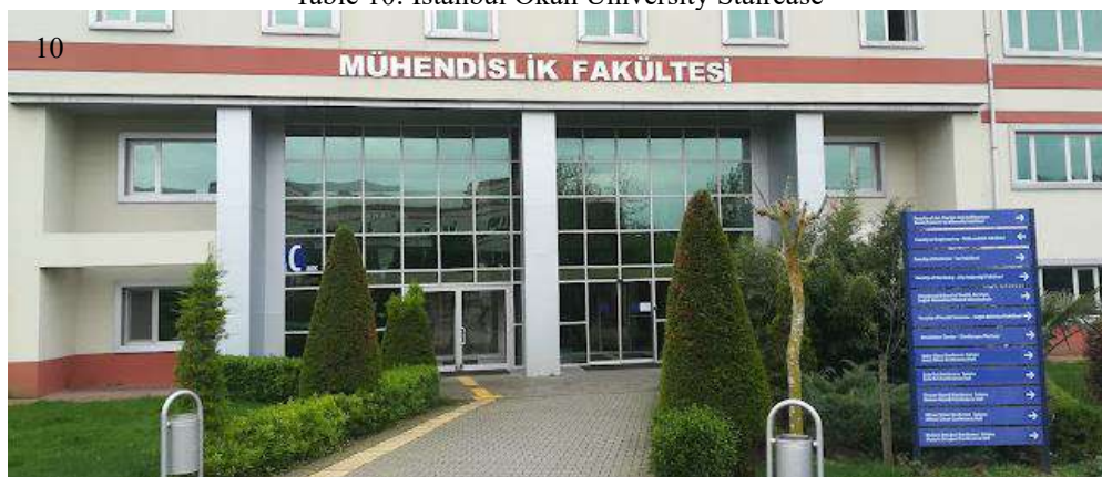
Figure 14: İstanbul Okan University Entrance to the College of Engineering building
