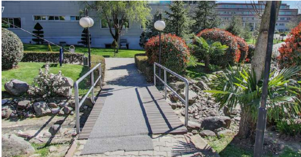
Figure 11: İstanbul Okan University A pedestrian walkway 2
