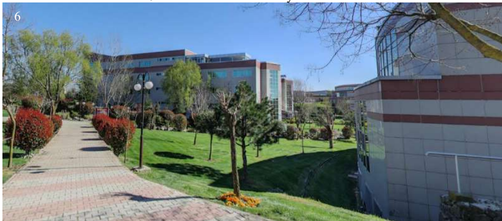
Figure 10: İstanbul Okan University A pedestrian walkway
