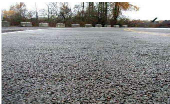
Fig 1. Permeable Concrete Road
