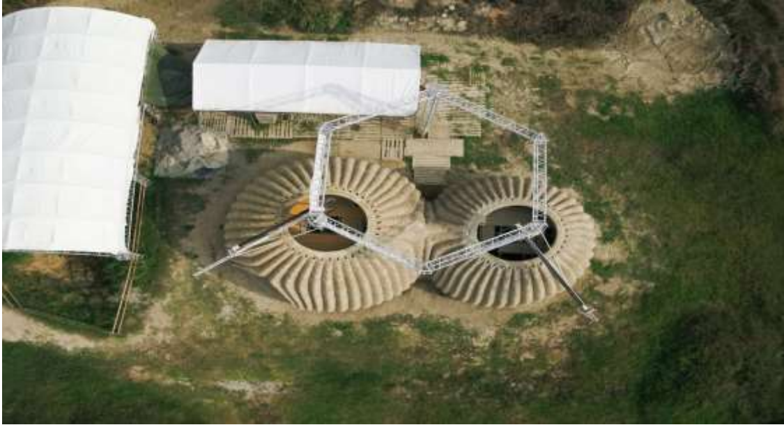
Fig.6 The prototype was developed as a response to climate emergency. Photograph is by Italdron
