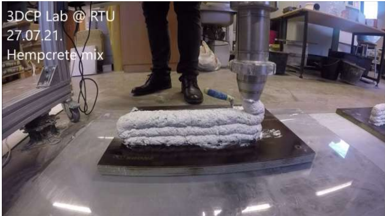
Fig.10 A 3D-printing robot puts down layer-upon-layer
