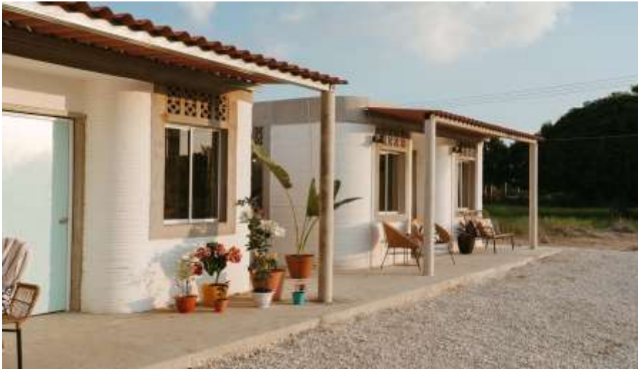
Fig.1 The first two 3D-printed homes in Tabasco sit side by side on Lavacrete
