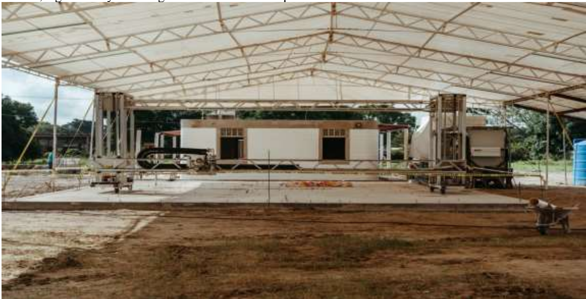
Fig.2 ICON's Vulcan II printer prints homes atop a cement pad.
