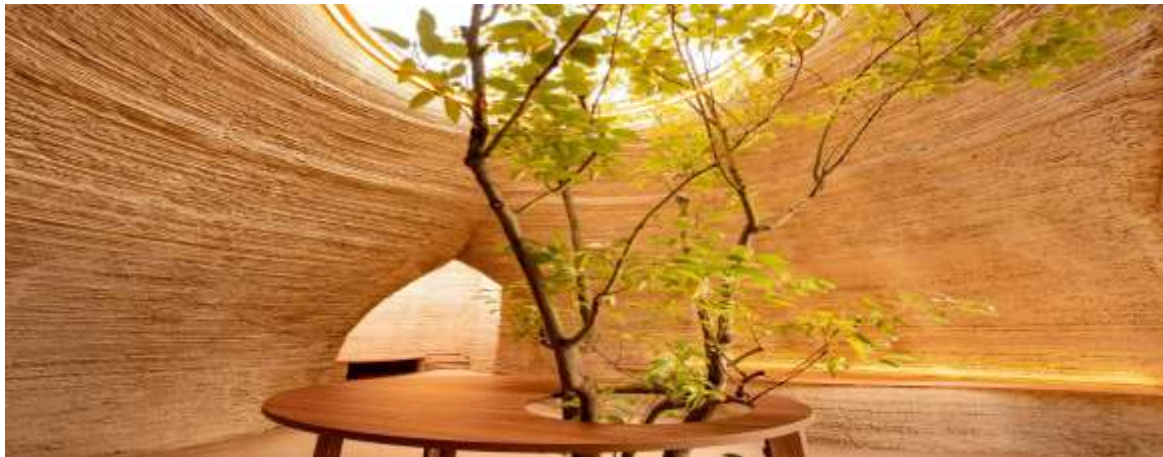
Fig.8 The prototype was printed using 350 layers of clay
