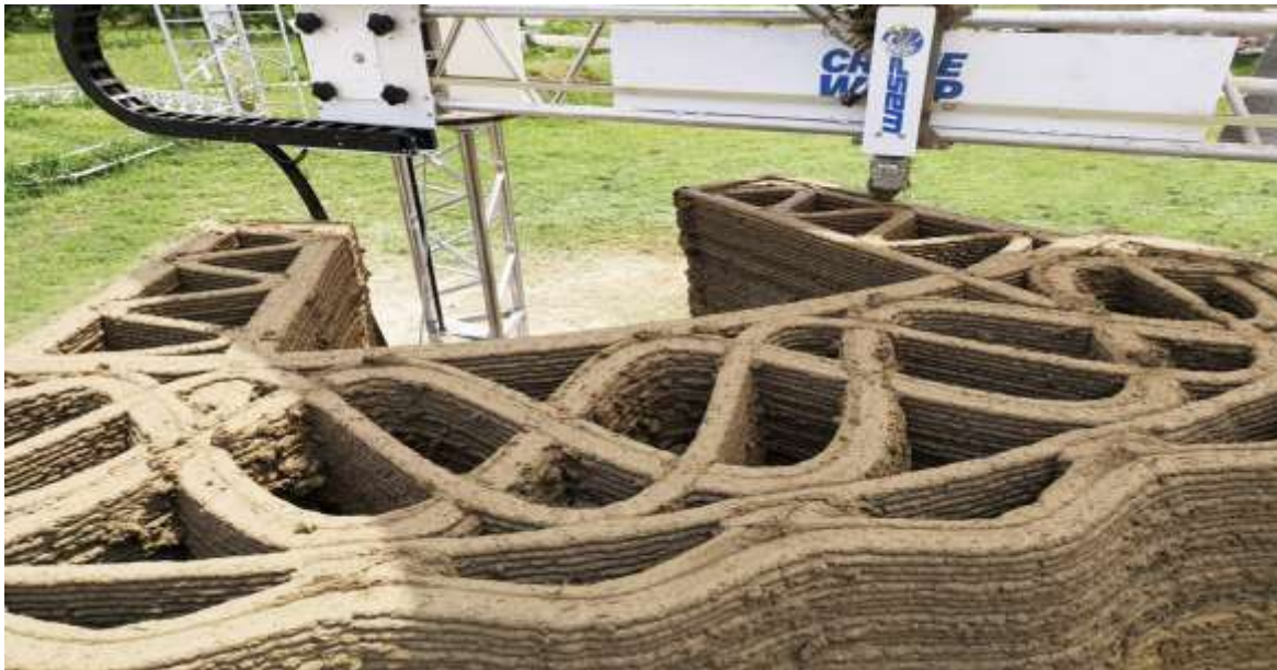
Fig.5 Undulating curved layers provide structural stability
