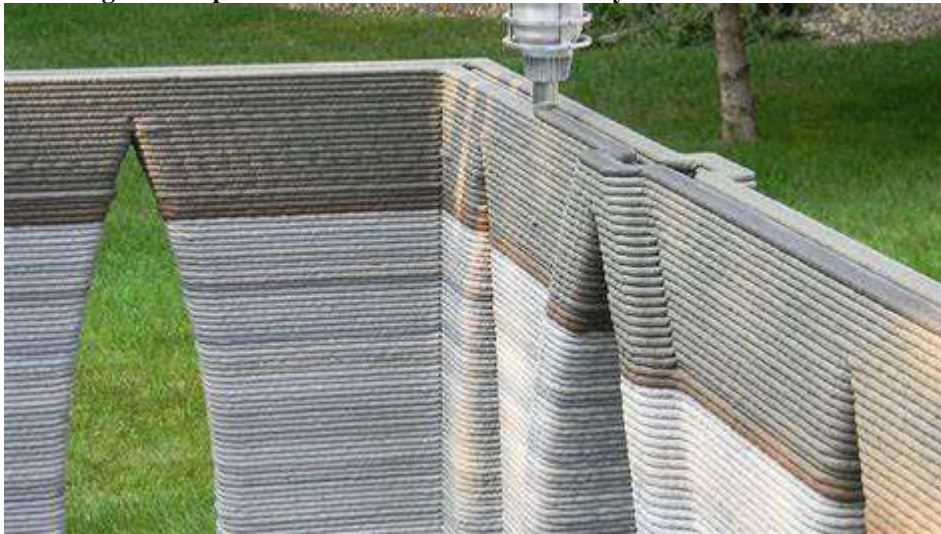
Fig.(8) 3D printing bulding - Bing This is the world's first 3D printed hotel.
