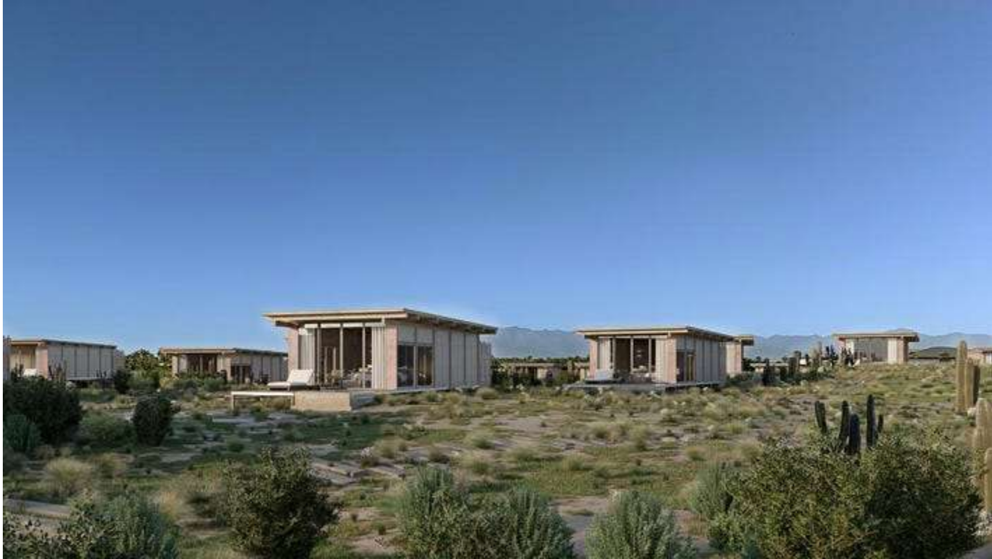
Fig.(15) A view of the buildings
