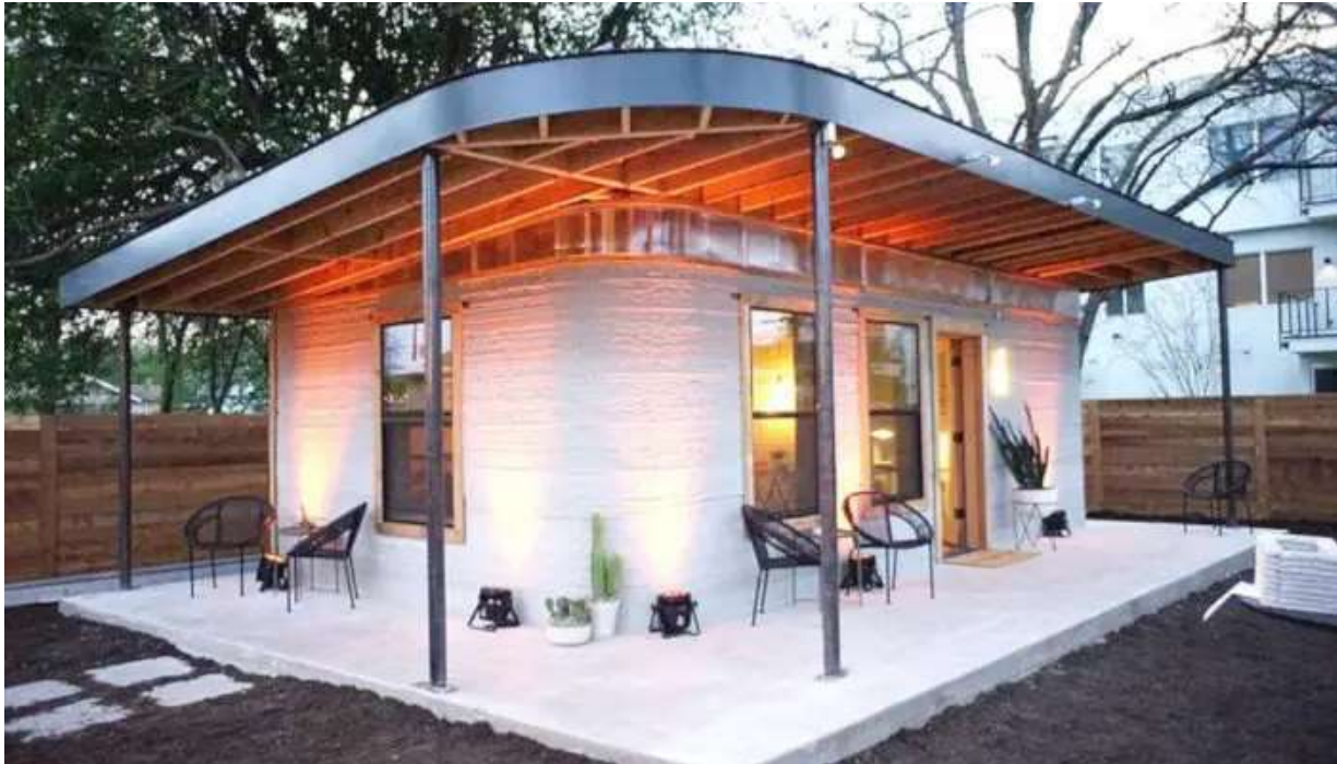
Fig.(5)3D printed house cost: $10,000 Located: USA The 12 Most Exciting 3D Printed House Builds 2022 - 3DSourced
