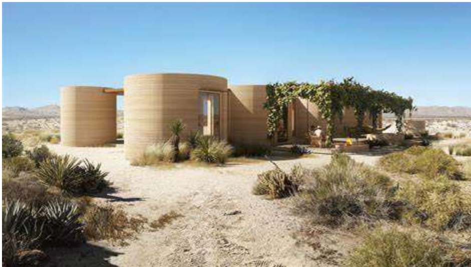
Fig.(16) A view of the buildings
