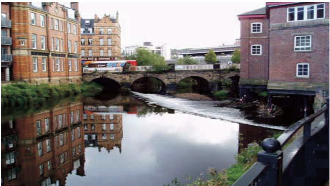
Figure 1.1: The squeeze on the River Don Source: Environment Agency, 2007
