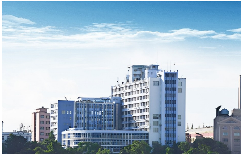
Photograph 2: The New Secretariat Building
