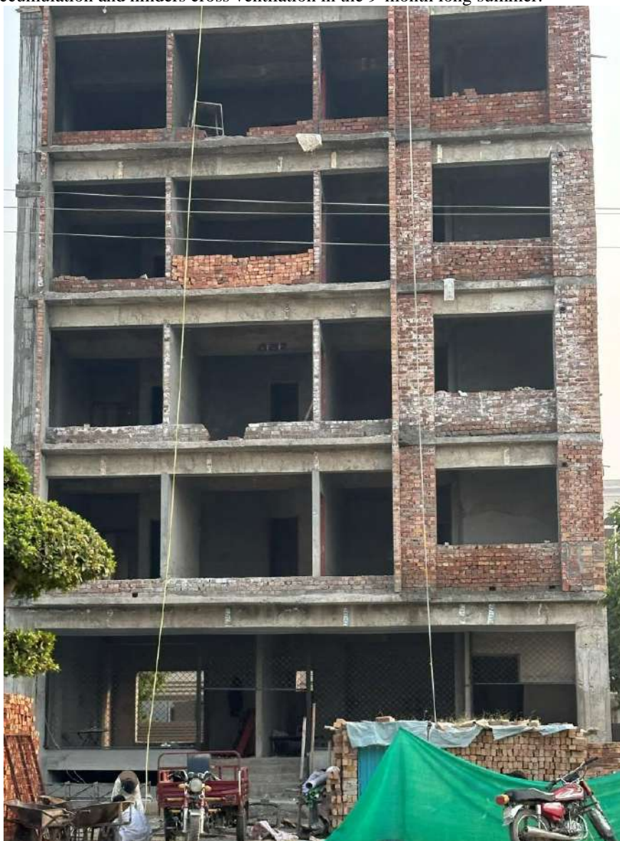
Figure 4 Recent low rise apartment building construction in Lahore
