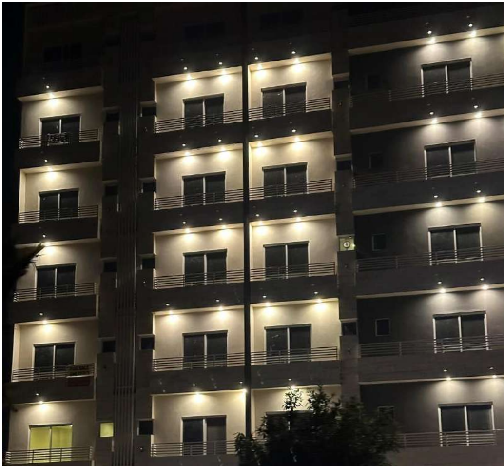
Figure 6 Recently built low-rise apartment building in Lahore. The balconies do not allow free moving space for the resident to leisurely sit and have family time as a source of outdoor activity, such a balcony barely even serves as an outdoor space. Taken by Author 2023
