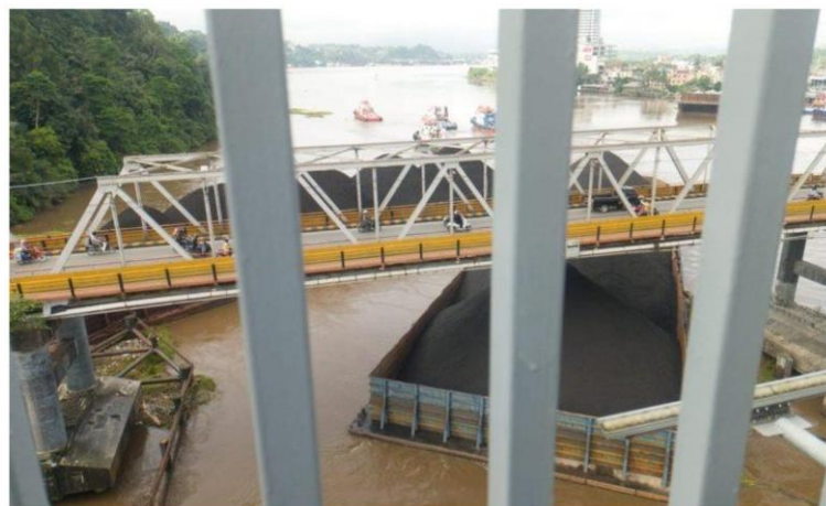
Figure 4. post-collision situation on Mahakam-1 Bridge
