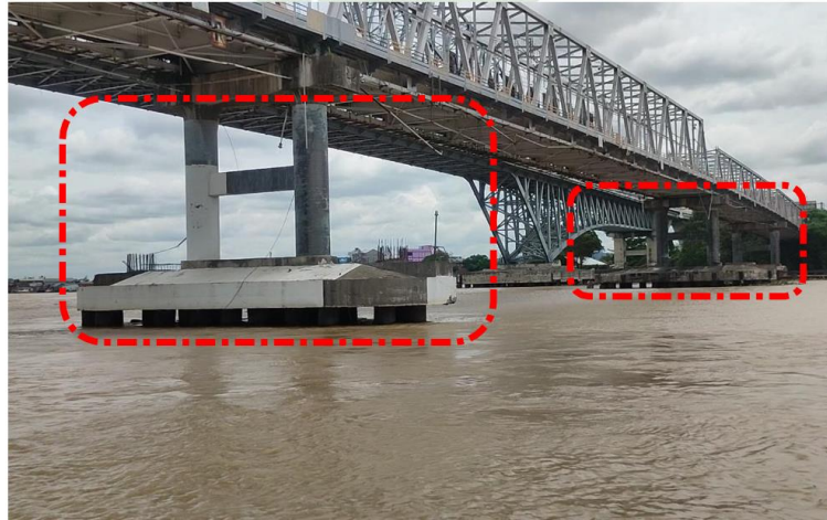
Figure 3. Pillars and fenders of Mahakam Bridge-1
