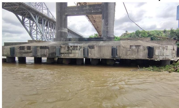
Figure 9. Fender installation condition on pillar P4
