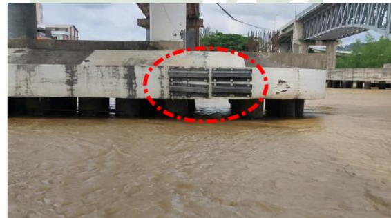
Figure 8. Fender installation condition on P3 pillar at downstream river position
