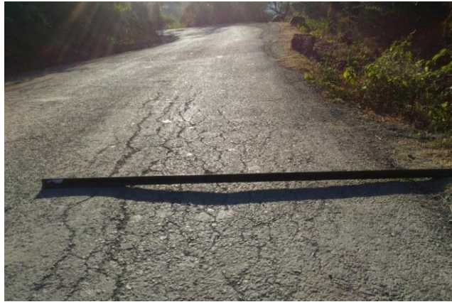
Fig. 2: Rut Depth/Rutting
