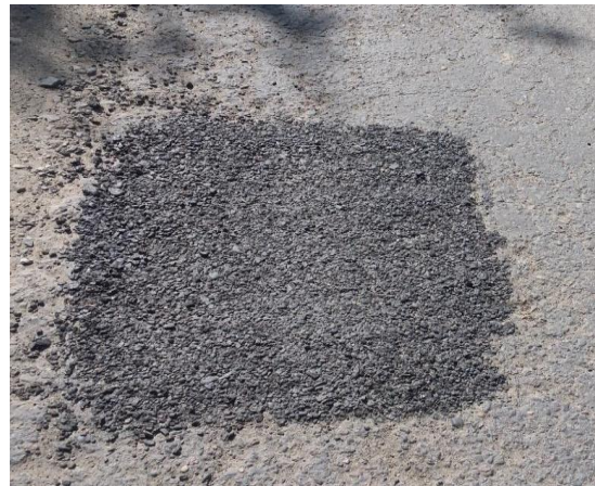
Fig. 4: Patching at RR-1
