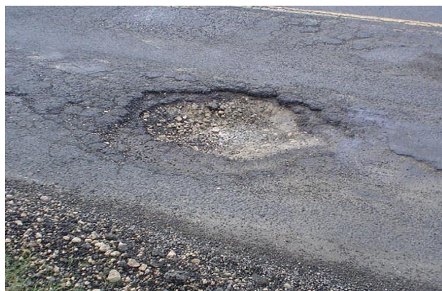
Fig. 3: Pothole Depression
