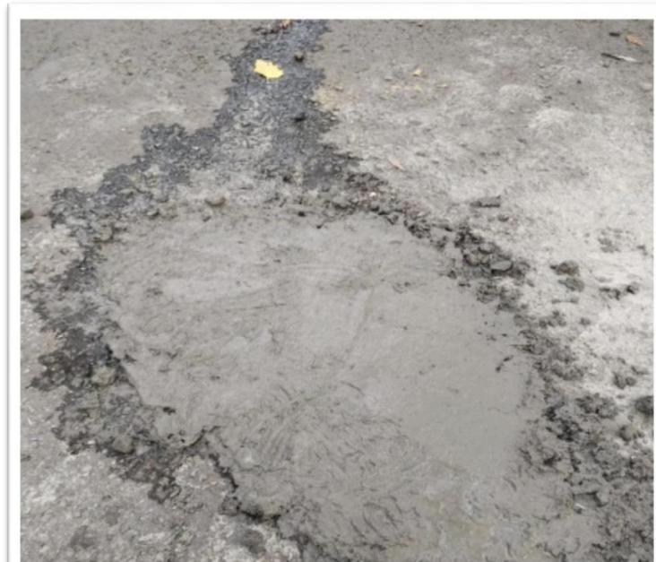
Fig 4 Patch Filling
